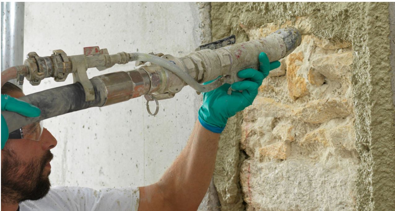
Parnatur® is easy to apply with a standard spraying machine
