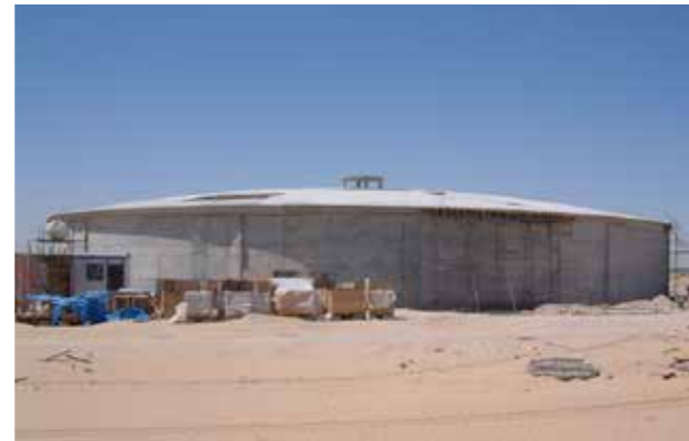
AL AJBAN WATER RESERVOIR, ABU DHABI, U.A.E. 2003
