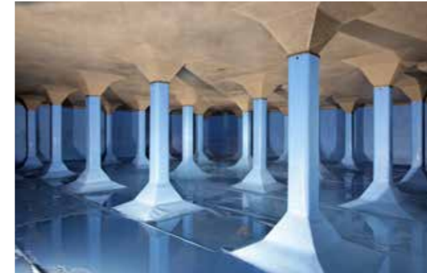
WATER RESERVOIR LUDWIGSBURG, GERMANY 2011
