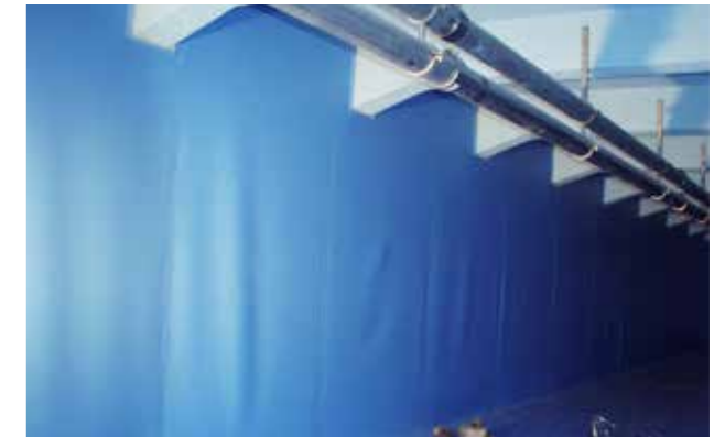
WATER RESERVOIR ZOLLERNALB, GERMANY 2006
