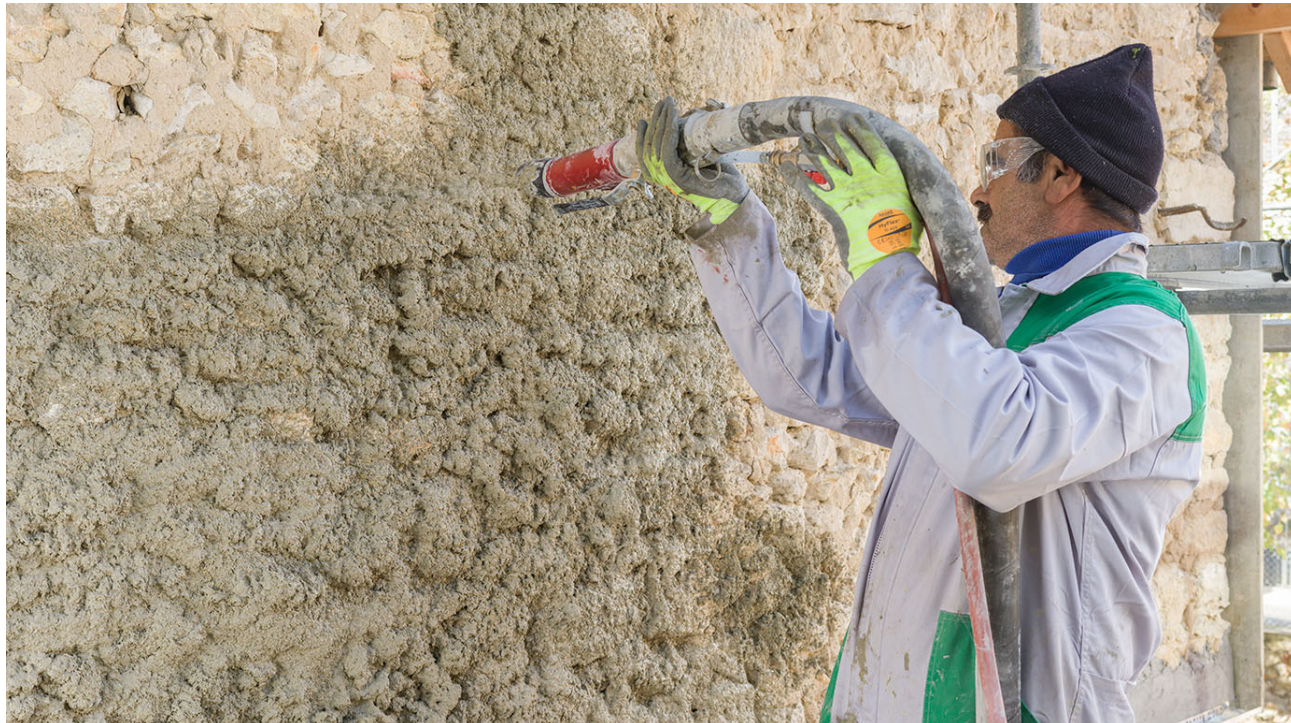
PARNATUR®, the first “easy-to-spray” thermal and phonic insulation hemp-based mortar
