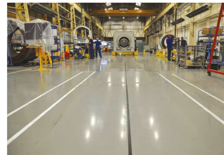
Durability, ease of cleaning and wayfinding provided by Sikafloor® in a cargo handling facility.
