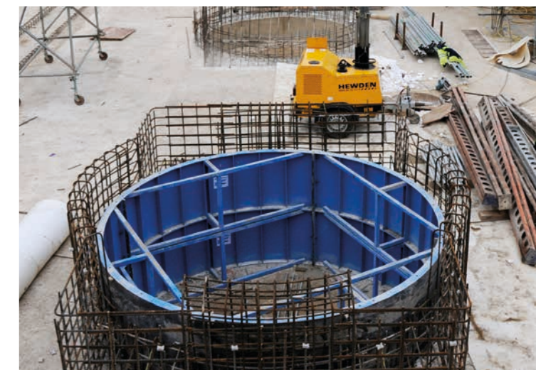
Fuel pumping station - Sikagard® protective coatings.
