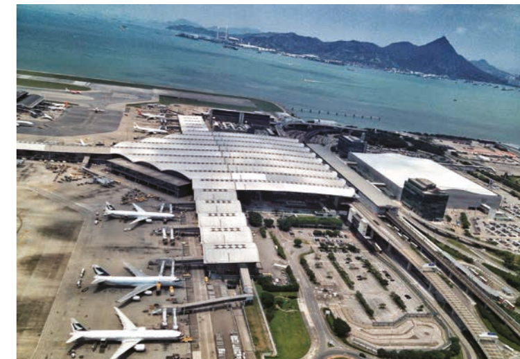
Sika Sarnafil® single ply roofing membrane on the main terminal building at Hongkong International Airport.
