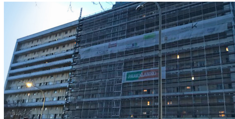
Le Moustoir jobsite in France.
