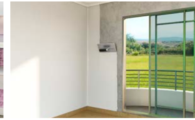
INTERIOR WALL LEVELING & FINISHING
