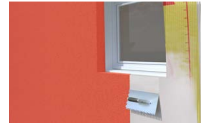
EXTERIOR WALL LEVELING AND DECORATIVE FINISHING
