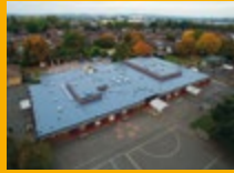
LIQUID APPLIED ROOFING
