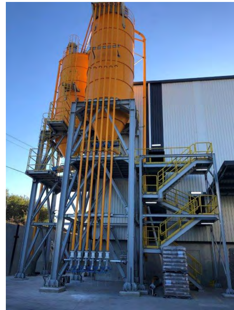
New mortar plant Australia.
