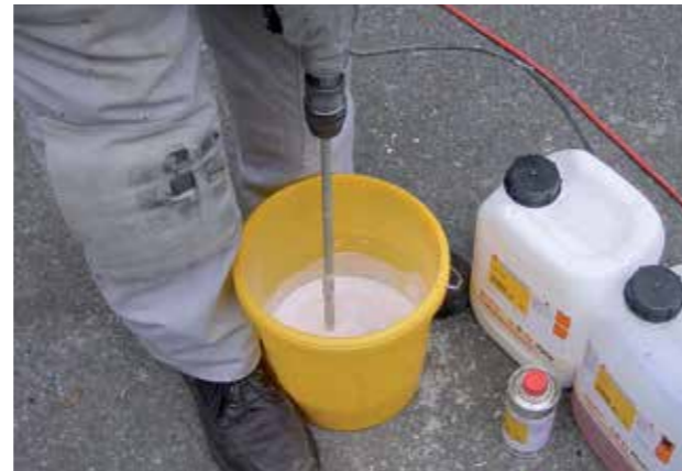
Mixing of an acrylic based Sika injection resin
