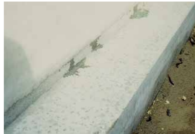
Simple injection process on site
