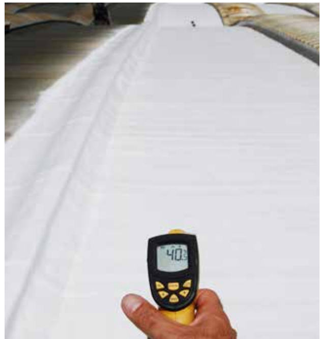
Roof temperature after LAM application.
