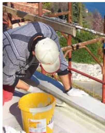
Detailing on bituminous membranes
