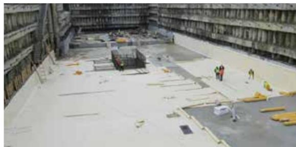
Vertical excavation wall, typically use for SikaProof® A under the raft and at the walls.
