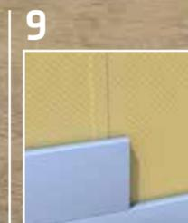
9 WT protection sheet/felt and thermal insulation boards
